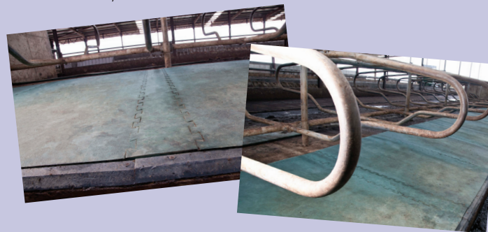
2 sided interlocking mats with fixing strip at the back of the cubicle
