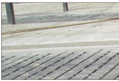
■ ABOVE: Double tank with four pieces 1.9m end to end of Durapak Slatted Rubber.
